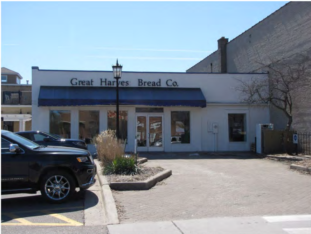
Main East 139_Looking South
