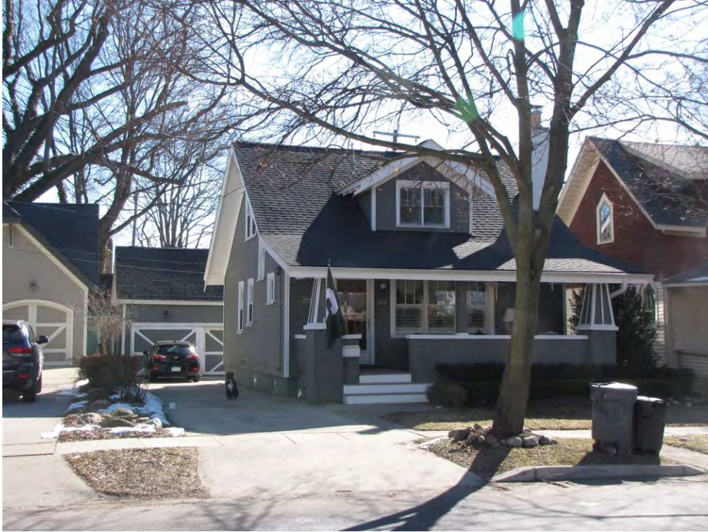
Wing North 214_Looking Southeast
