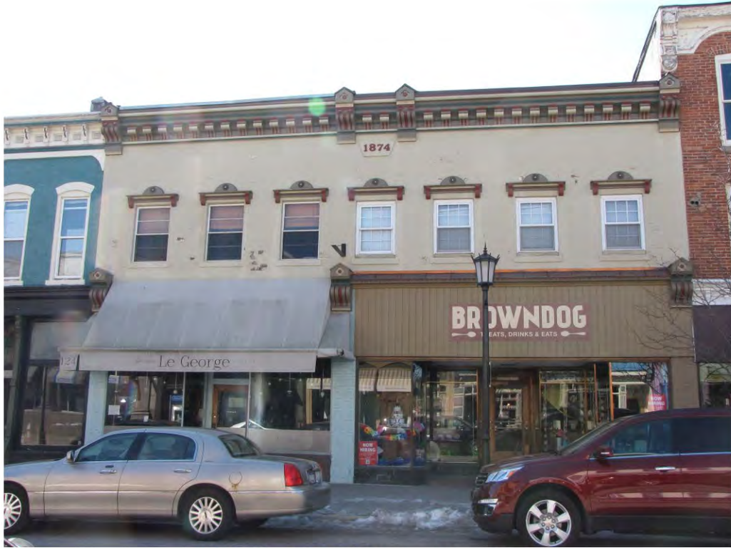
Main East 120-124_Looking South
