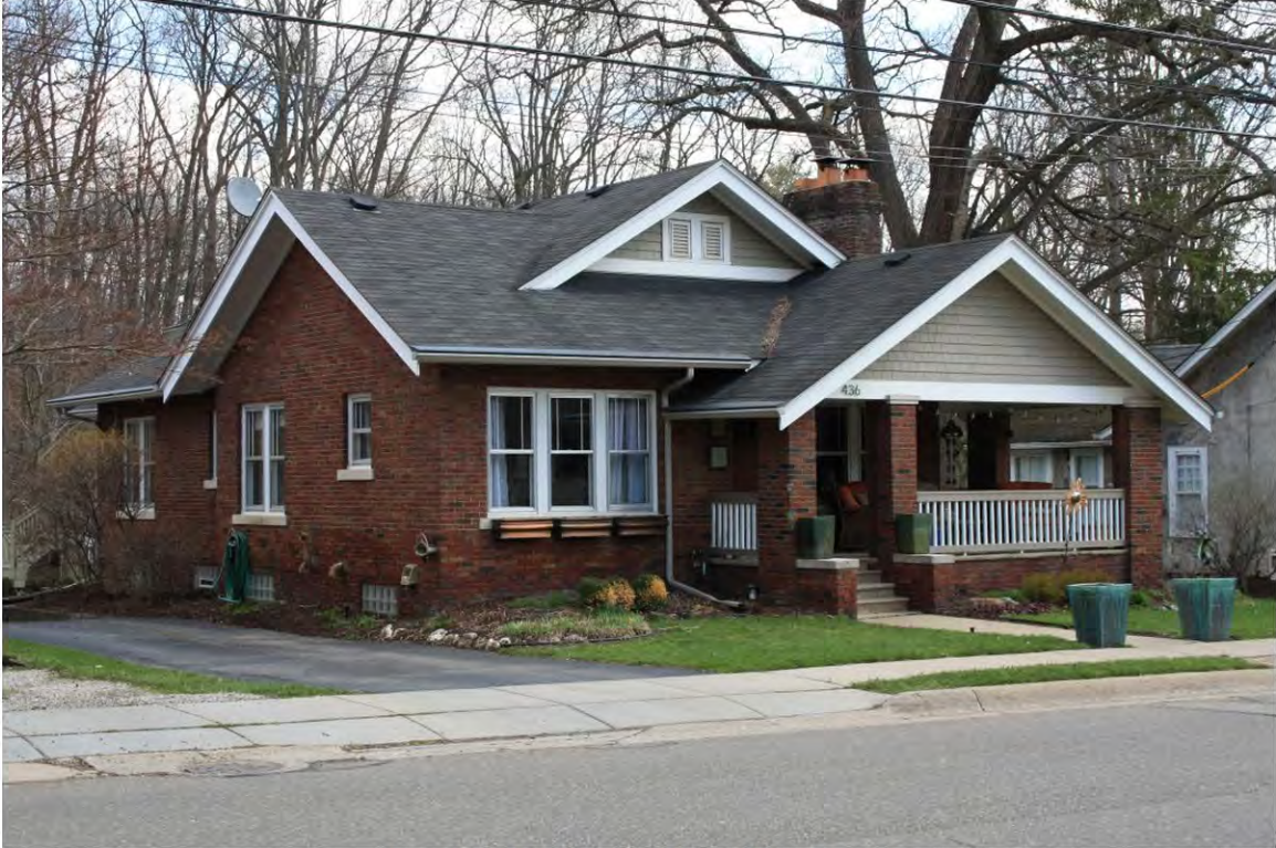
Randolph 436_Looking Northeast
