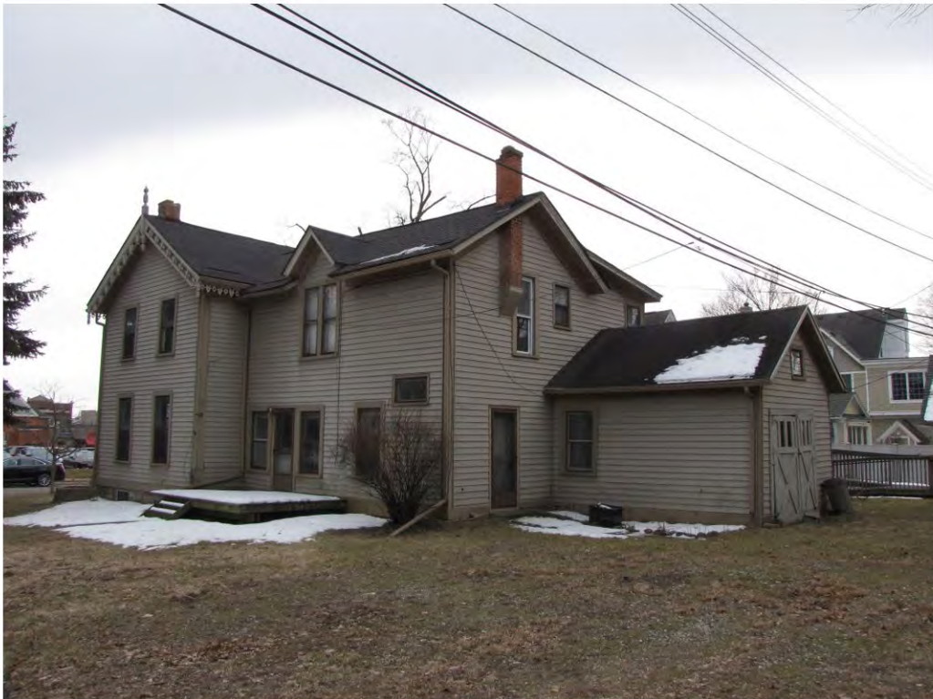
Wing North 129_Looking Southeast
