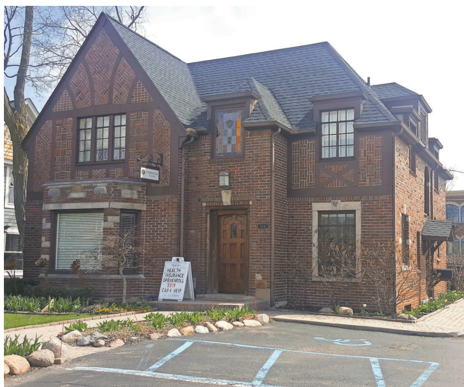
324 Main St. is a great example of the Tudor style, with its asymmetrical design, prominent cross gable, decorative brick and large bay window.
