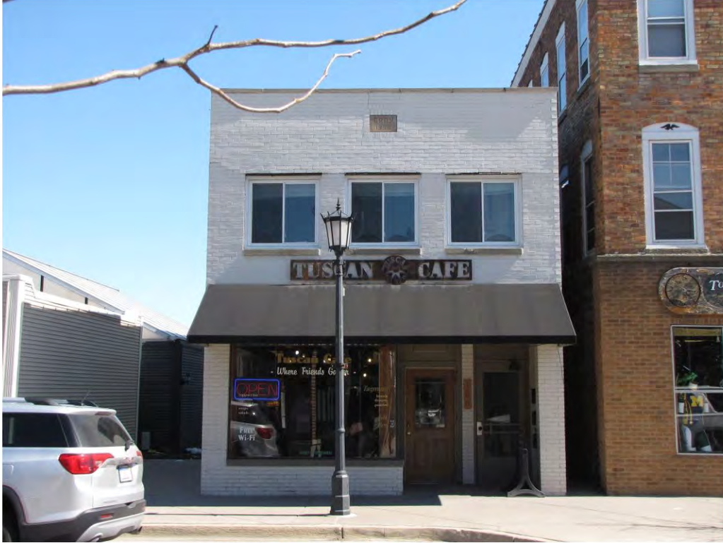
Center North 150_Looking East
