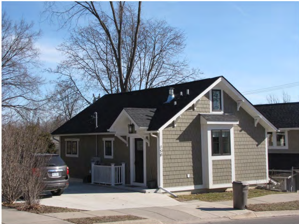
Randolph 108_Looking Northeast
