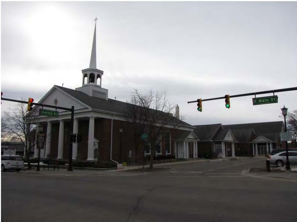
Main East 200_Looking Southeast
