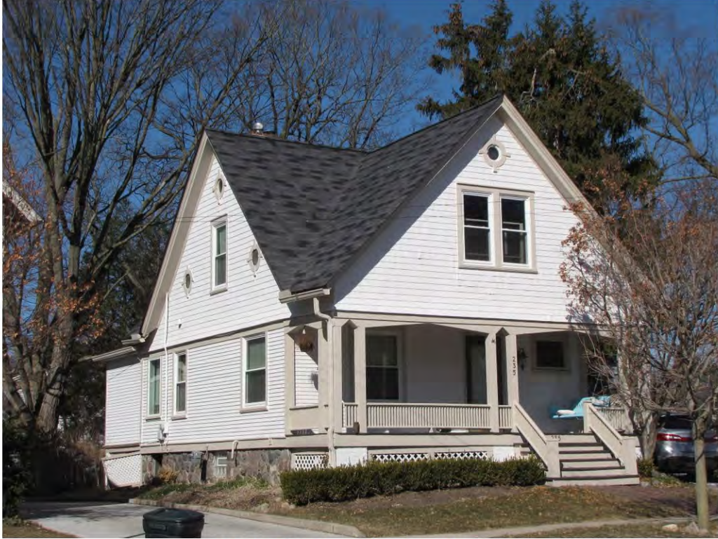
High 235_ Looking Northwest
