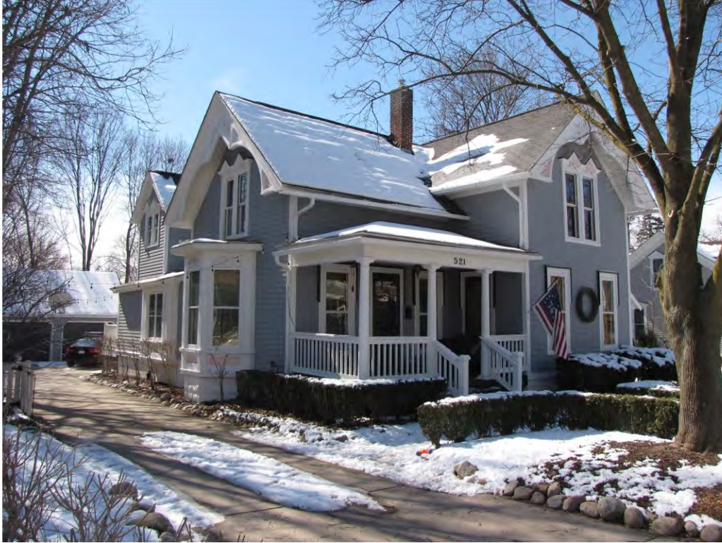
Main West 521_Looking Southwest
