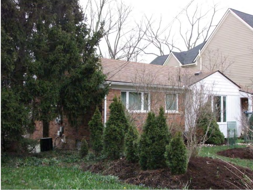
Rogers North 368_Looking Southeast
