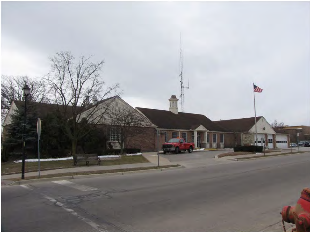
Main West 215_Looking Southwest
