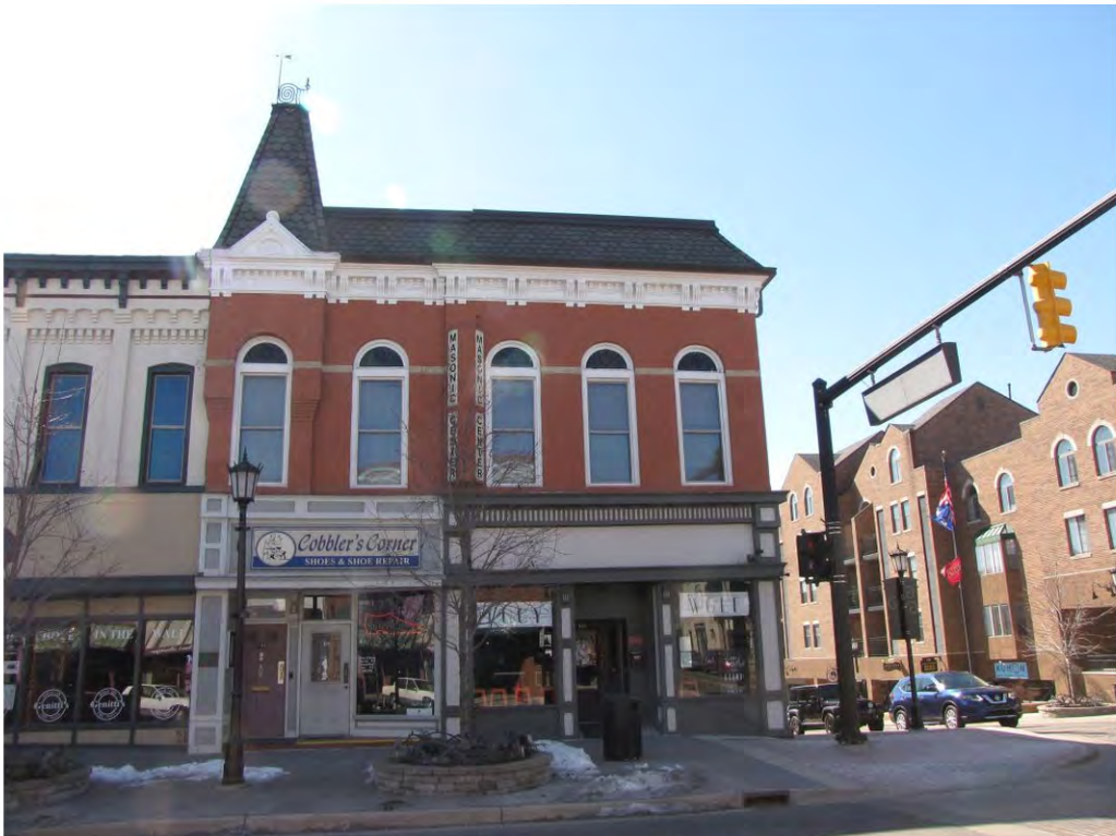
Main East 102-106 and Center South 113_Looking South
