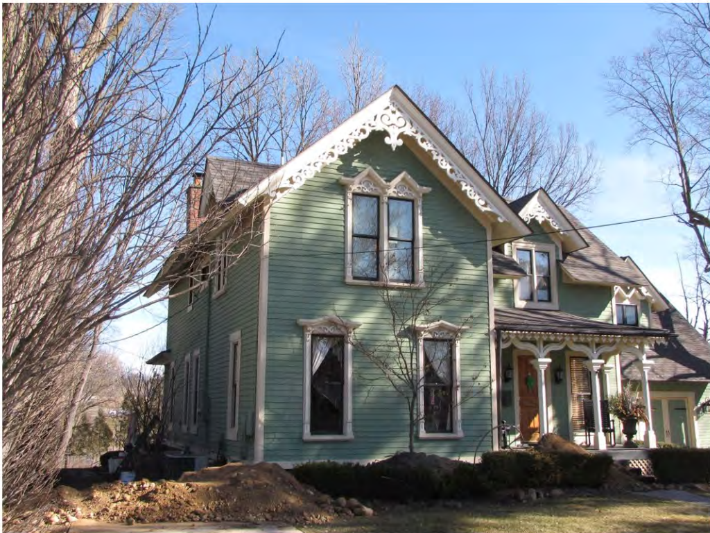
Randolph 124_Looking Northeast
